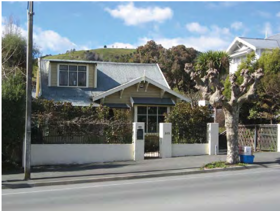
Figure 32: Collingwood Street frontage with a low solid wall and a highly visually permeable fence above with planting providing partial screening while maintaining a visual connection. The effect is successful.
