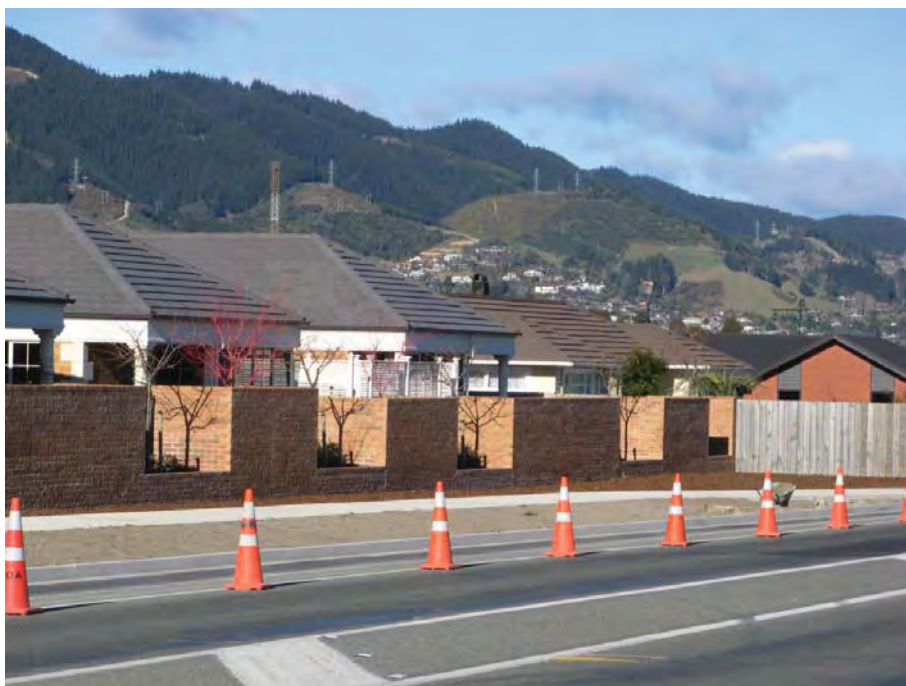
Figure 16: Main Road Stoke: contrast of a high fence which allows views to and from the street, with a blank, close boarded fence
