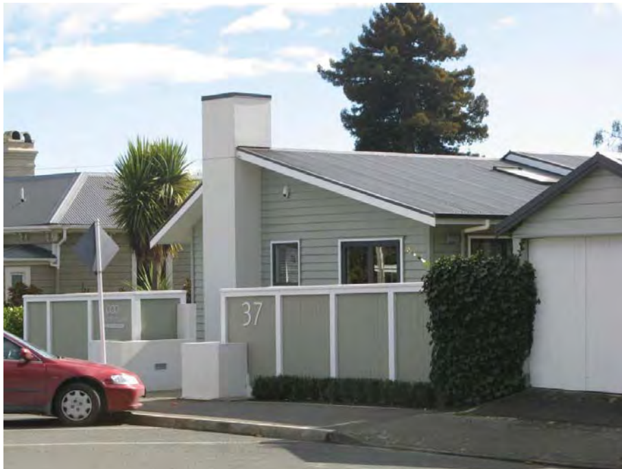
Figure 18: 37 Manuka Street: a well-designed high front fence, benefitting from a wide opening at the centre, careful aesthetic integration of fence and buildings, setbacks and planting and a wide opening at the centre.
