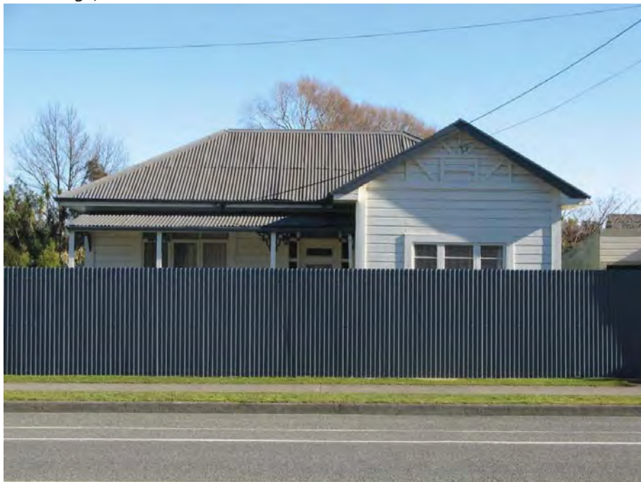
Figure 6: 50 Muritai Street Tahunanui – a character cottage compromised by a high fence
