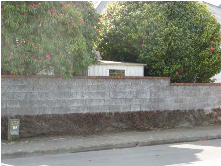
Figure 21: High concrete block wall to east of 37 Manuka Street frontage
