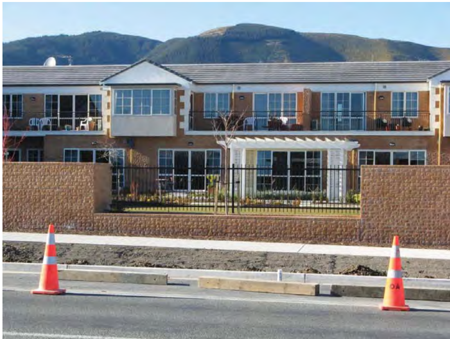
Figure 15: Retirement Village, Main Road Stoke demonstrating how a combination of closure and openness can be achieved.
